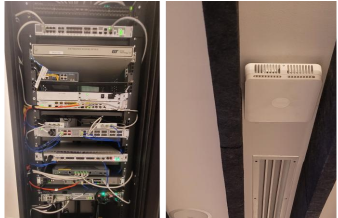
Fig. 2. Indoor 5G AS architecture utilized to connect the industrial devices during the tests.
