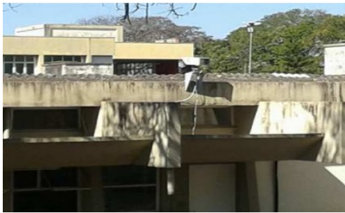
Fig. 2. View of the receiver installed on the roof of a building.
